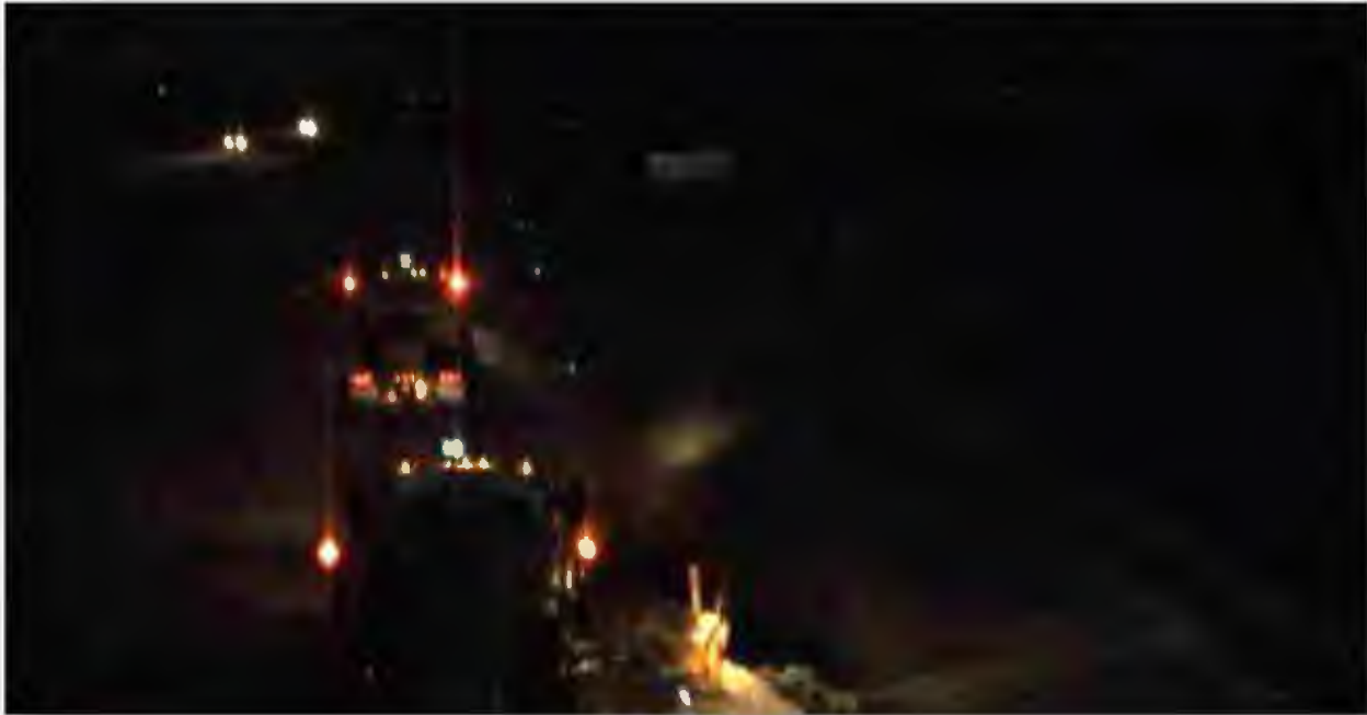
LEDline® Being Snow Ploughed on The Ontario 403 Freeway: (The picture taken from a video in a major storm).
